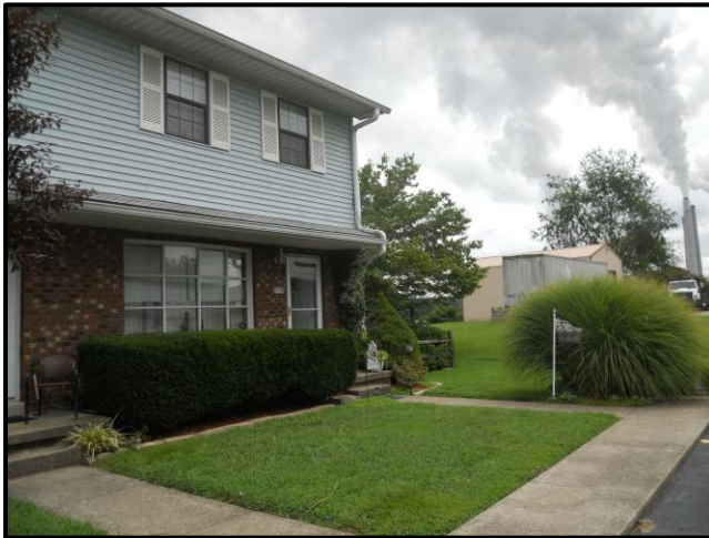
4-Remediated home, Nitro
